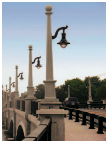
Lighting standards, Barrington and Warren Bridges, RI
