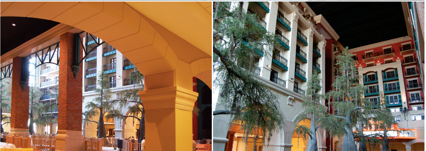
Fiberglass Ornamentation for entire atrium interior, buildings, trim and facades, Paragon Casino Resort atrium complex, Marksville, LA
