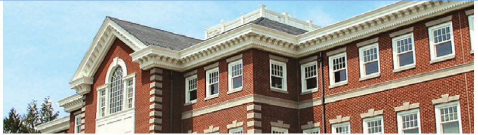
Red Cross Office Building, New Brunswick, NJ
