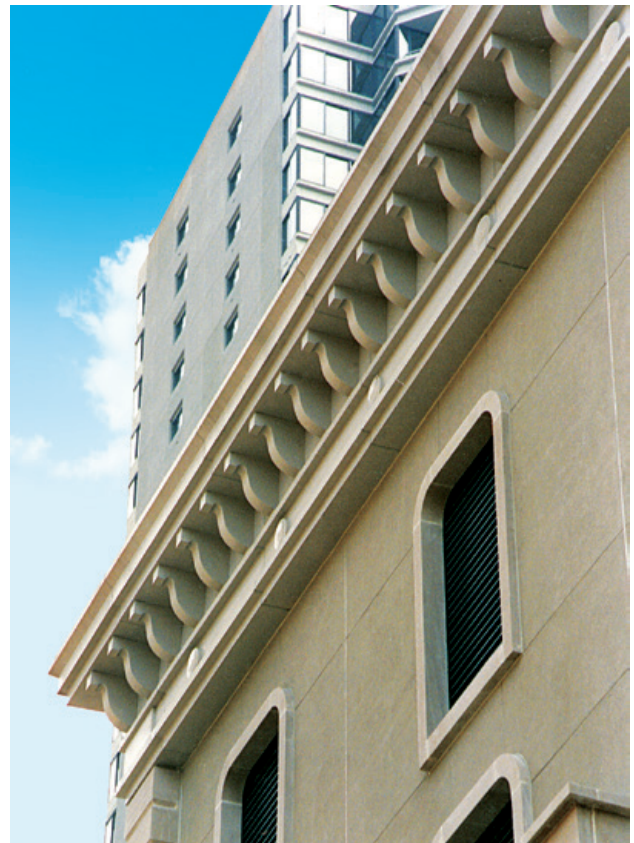
Rittenhouse Parking Garage, Philadelphia, PA
