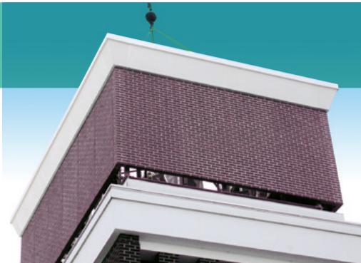
Verizon Communications, Paoli, PA
