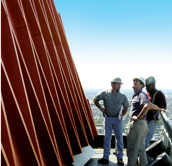
350 feet above ground, custom fiberglass panels (50'L x 24'H)
