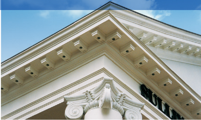
Sullivan County Court House, Blountville, TN
