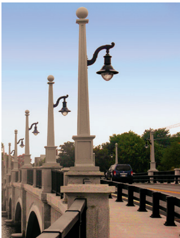
Lighting standards, Barrington and Warren Bridges, RI
