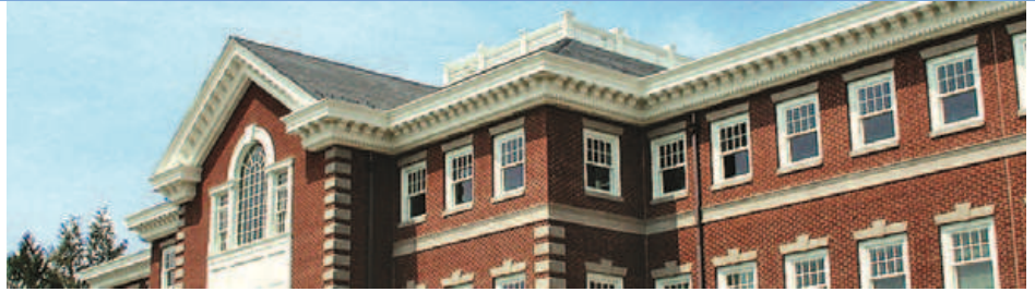
Red Cross Office Building, New Brunswick, NJ
