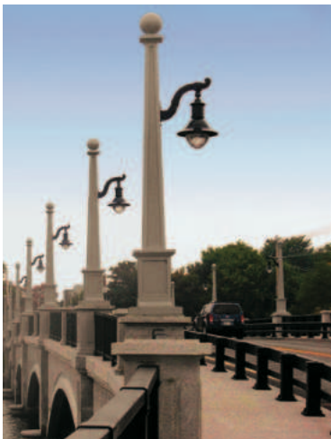
Lighting standards, Barrington and Warren Bridges, RI
