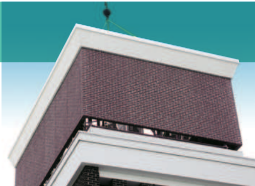
Verizon Communications, Paoli, PA
